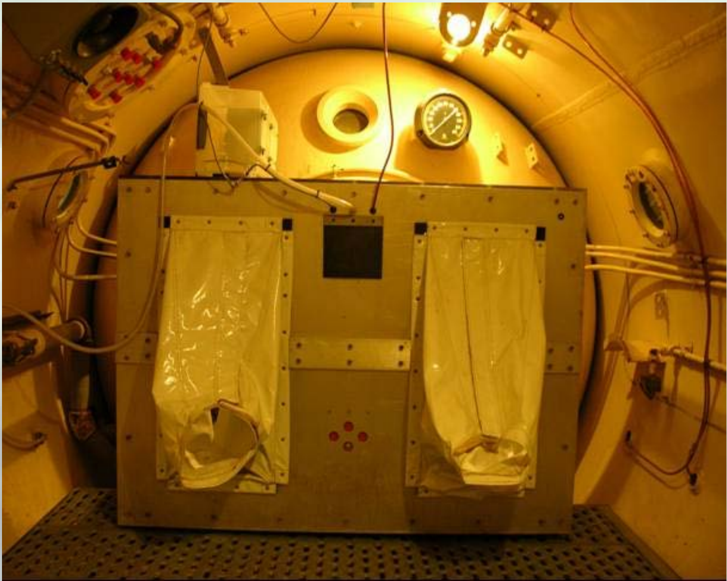
Figure 1. UW O 2 delivery system used to evaluate emergency decompression to surface pressure.
